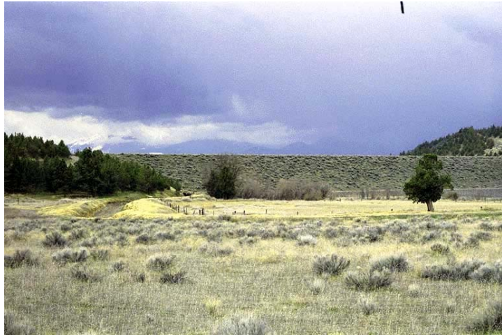
Figure 4. Dwinnell Dam looking south with the canal at left into which almost all flows from the reservoir are diverted. Photo from KRIS Version 3.0 (TCRCD, 2003).
